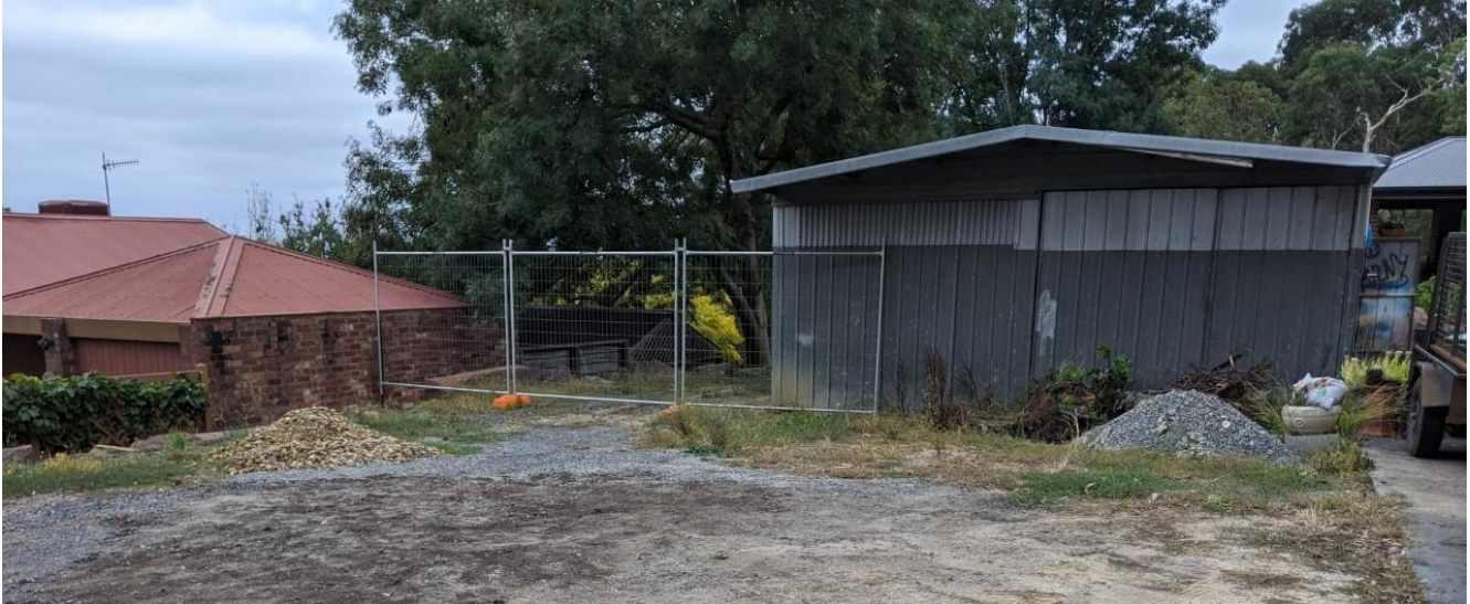
Figure 1. Existing shed (Tapir, 2022)
